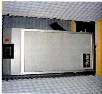
Parker nitrogen compressor _____ RH control units RK2 _____ Pressure tank
